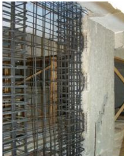
Construction Of RC Shear Wall
